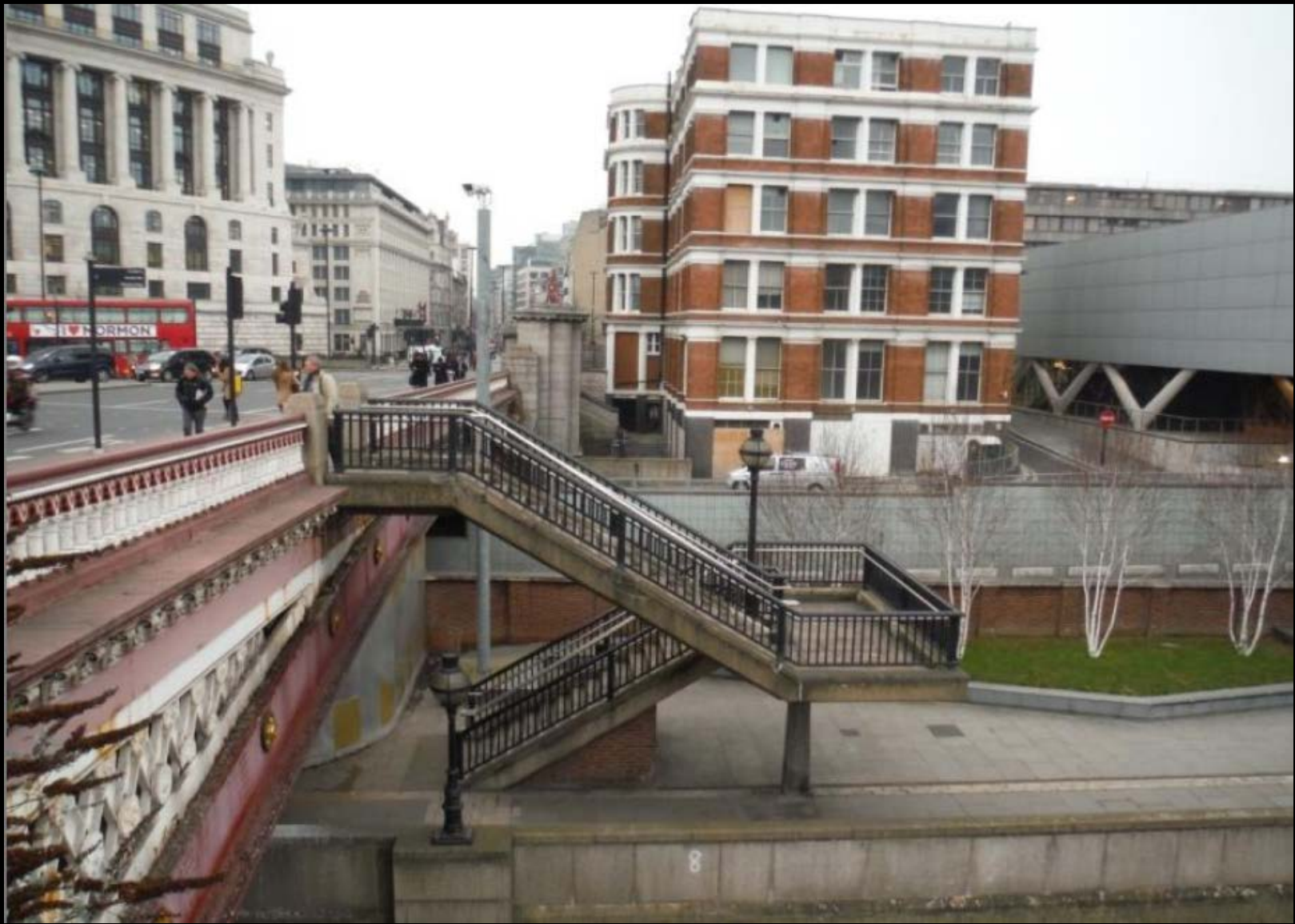
View north showing the southbound footpath on Blackfriars Bridge and the existing stairs to riverside walk
